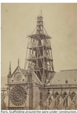
Paris, Scaffolding around the spire under construction, 1859 Photo attributed to the Broussin brothers
