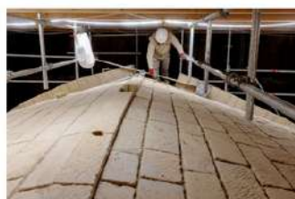
Paris, New vault dome of the cathedral, 2024 https://www.lesliefranklin.com/2024/04/15/paris-notre-dame-new-vault-dome/
