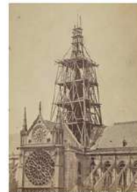
Paris, scaffolding around the spire under construction, 1859 https://www.lesliefranklin.com/2018/05/15/paris-notre-dame-scaffolding/
