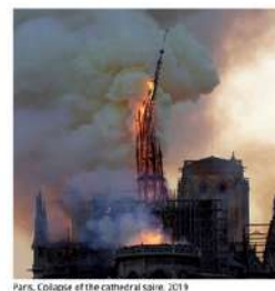
Paris, Collapse of the cathedral spire, 2019 https://www.lesliefranklin.com/2019/04/15/paris-notre-dame-collapse/
